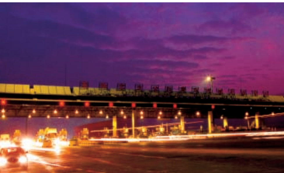
Beijing-Zhuhai Expressway (Guangzhou-Zhuhai Section)
