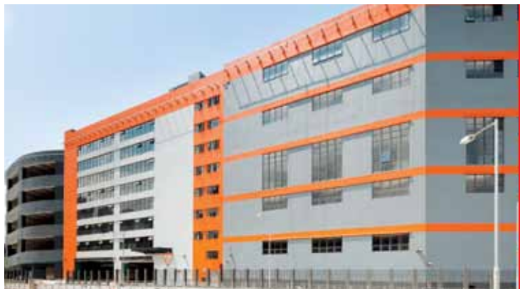
NWS Kwai Chung Logistics Centre
