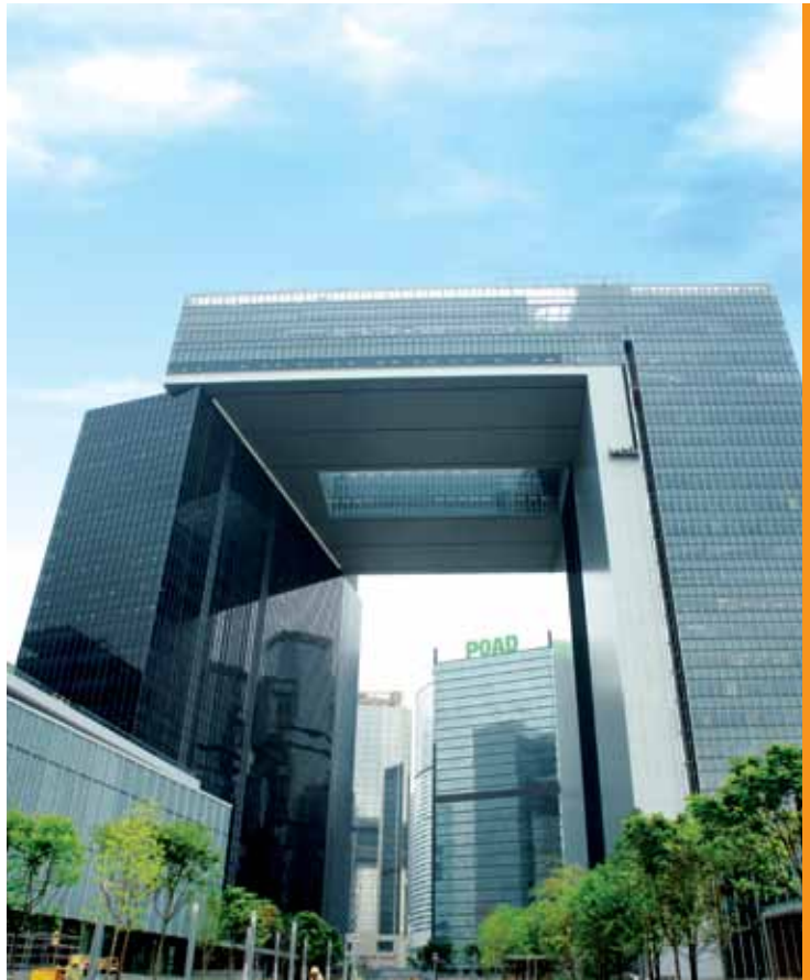
Tamar Development Project, a joint venture project with the participation of Hip Hing Construction
