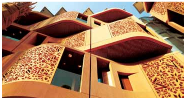
Masdar Institute of Science and Technology, Abu Dhabi, a project undertaken by Hip Hing Construction
