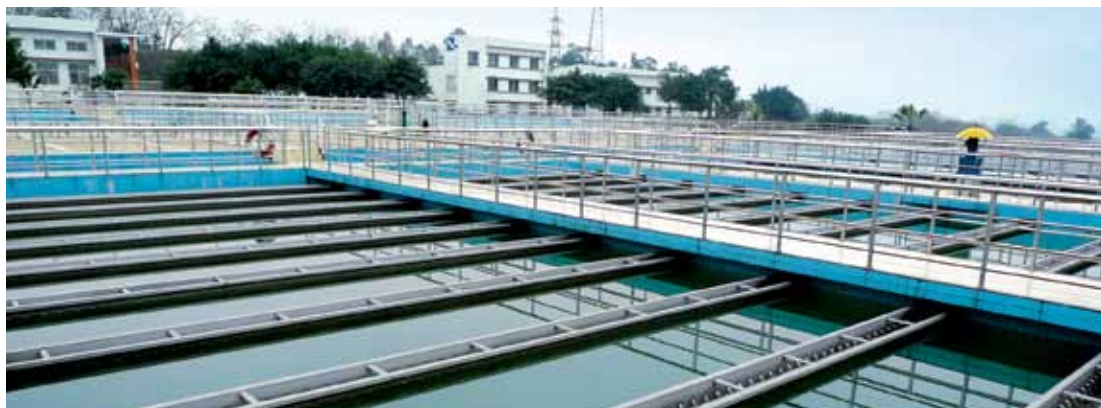
Chongqing Water Plant
