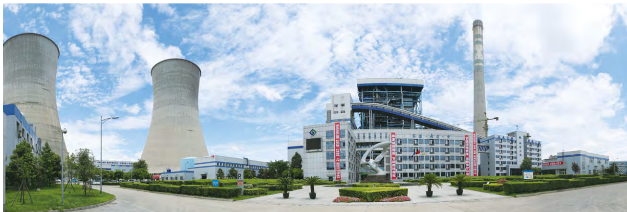
Chengdu Jintang Power Plant
