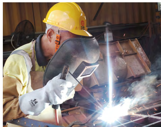
A Hip Hing construction worker in action
