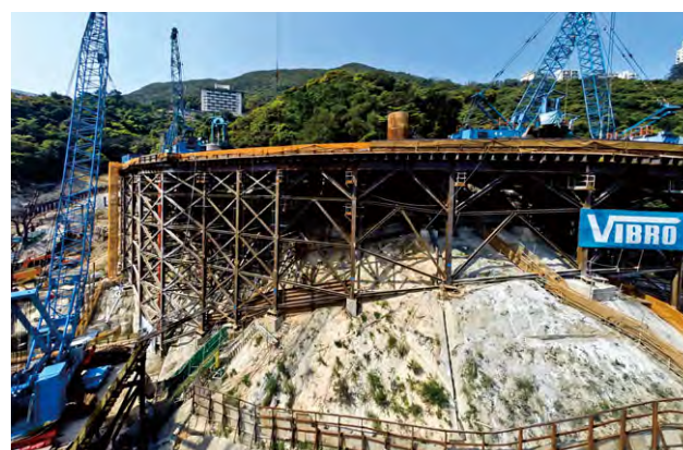
Piling and site formation works undertaken by Vibro (H.K.) Limited
