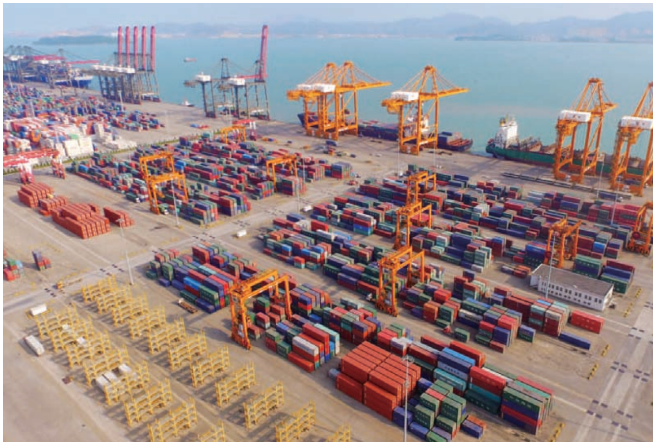
Xiamen Container Terminal
