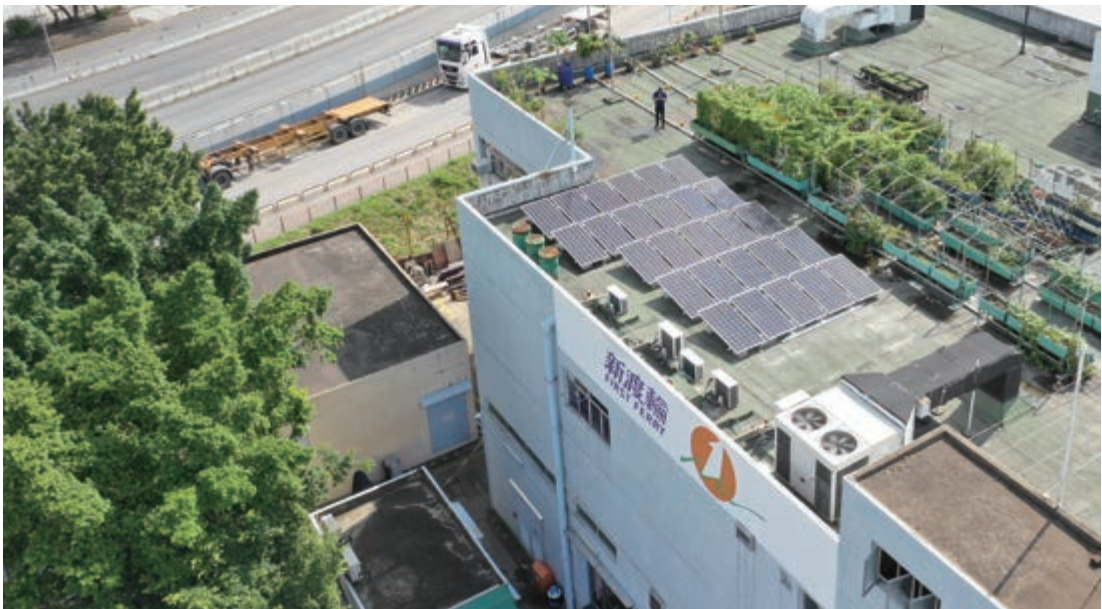
Solar panels on the roof of NWFF's office building in Cheung Sha Wan.
