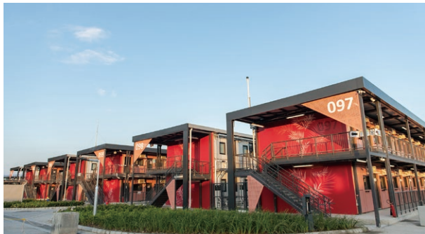
Temporary quarantine facilities at Penny's Bay
