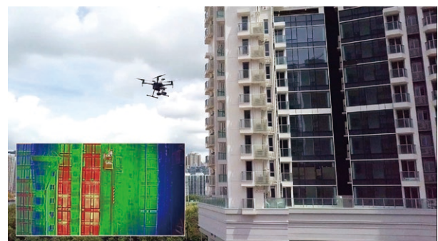
Applying drones and thermal imaging technique to manage on-site safety and quality in construction project
