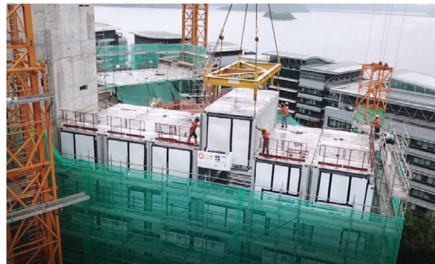
On-site installation of modules manufactured in factories
