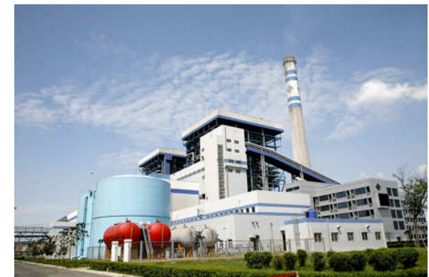
Chengdu Jintang Power Plant
