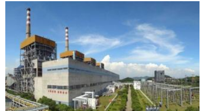
Zhujiang Power Plants
