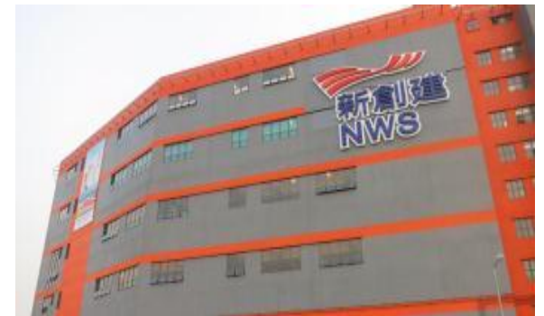
NWS Kwai Chung Logistics Centre
