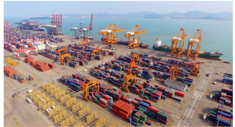
Xiamen Container Terminal Group
