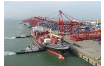
Xiamen Container Terminal Group
