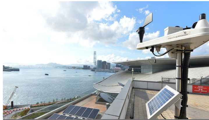
Installation solar power panels for feed-in tariff
