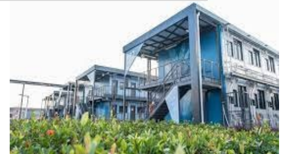
Hip Hing constructed 120 quarantine units
