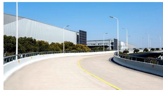
Ramp Access to Double Level
