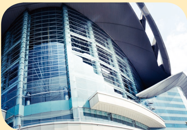
Heat-blocking film is installed on the largest glass window at HKCEC.
