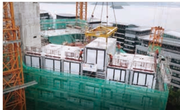
On-site installation of modules manufactured in factories
