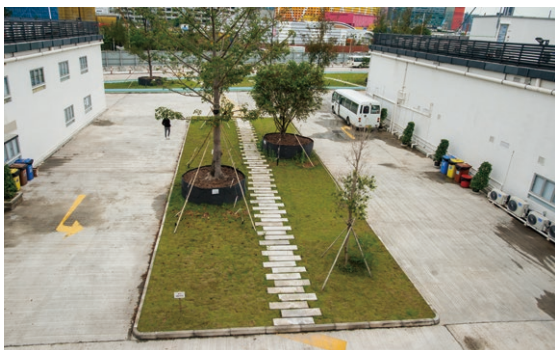
Protection of transplanted tree in construction site for future reinstatement
