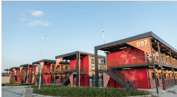
Temporary quarantine facilities at Penny's Bay
