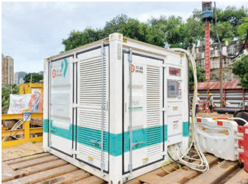
The BESS replaces the conventional diesel generators
